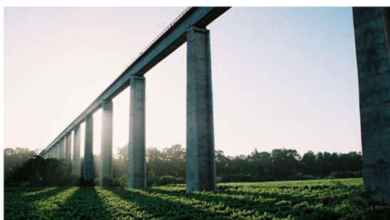
Sishen - Saldanha Railway Bridge over the Olifants River
